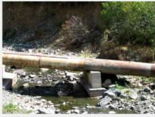
Yeghegis River in Pipes
