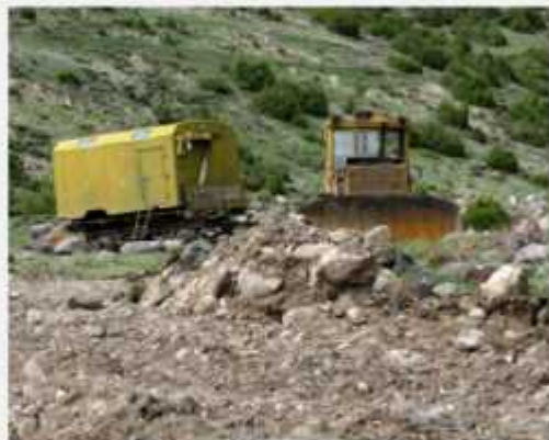
"Daranak" SHPP Construction
