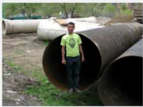
"Yegheg" SHPP Pipes
